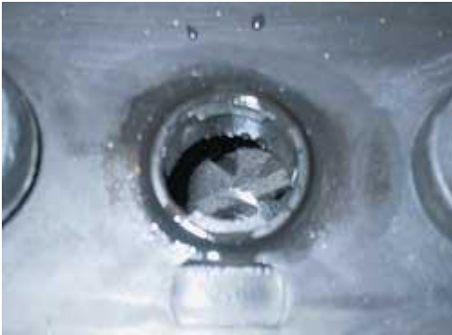
Looking into a lead-acid battery with the cap removed
